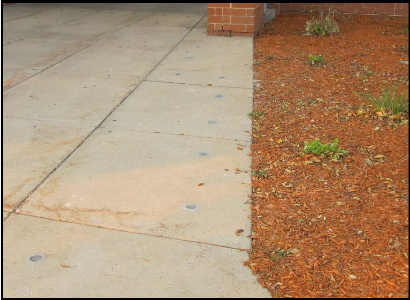
Same area after repairs
