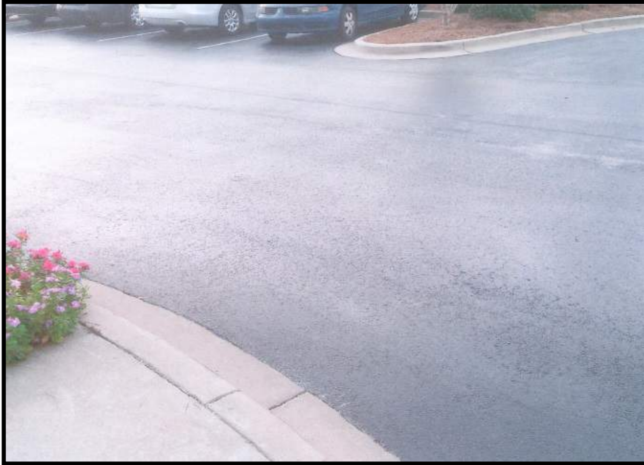
Motel Misstep – broken leg
